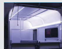
LED Internal Lighting
